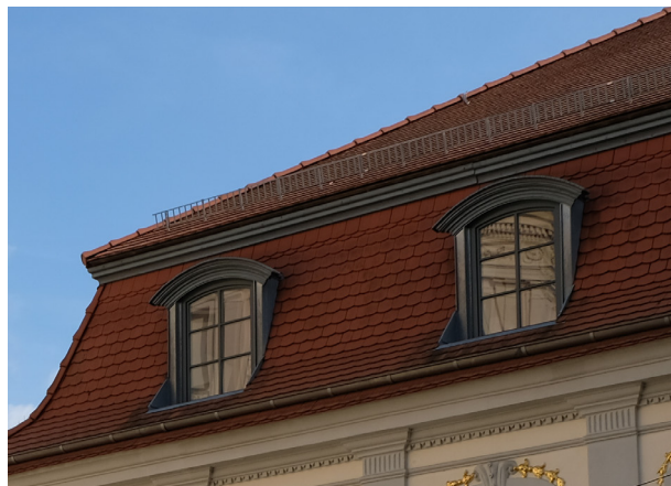
SANDOWER STRASSE Segmentbogengaupe
